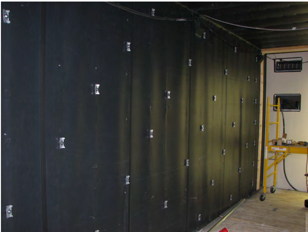
Low Frequency Absorption - 1Lb Vinyl Mass Barrier
