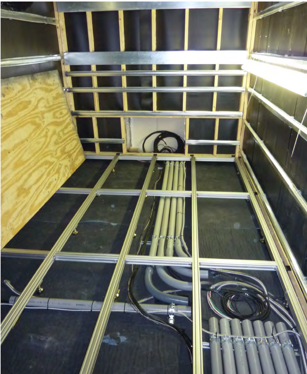
Floor Isolation - Suspended aluminum structure with Quiet Liner Acoustic Sound Sealant on all edges and corners.
